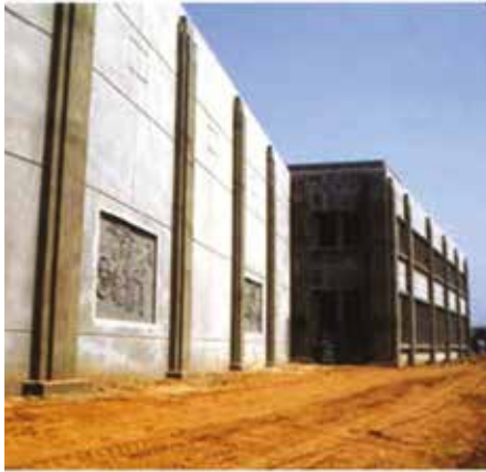
In addition to the smoothly patched tilt-up concrete panels, the building features integrally cast bas-relief sculptures that are textured with a fine sandblast finish.
