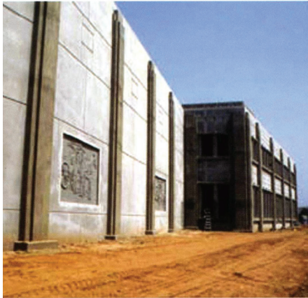
In addition to the smoothly patched tilt-up concrete panels, the building features integrally cast bas-relief sculptures that are textured with a fine sandblast finish.
