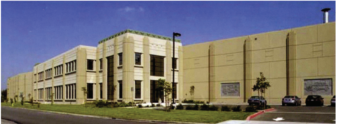
Art deco-inspired details and bas-relief concrete sculptures, along with ultra-smooth wall surfaces, show the aesthetic potential of contemporary tilt-up concrete construction. The Appfels warehouse building won an award in the recent Tilt-Up Concrete Association (TCA) competition for its "outstanding design and technical innovation."
