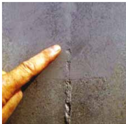
A new type of concrete patching compound allows smooth repair to concrete fins and defects that have been ground off. The compound can fill voids as deep as 12.7 mm (0.5 in.) in a single pass, yet it creates an even, featheredged transition into surrounding surfaces.
