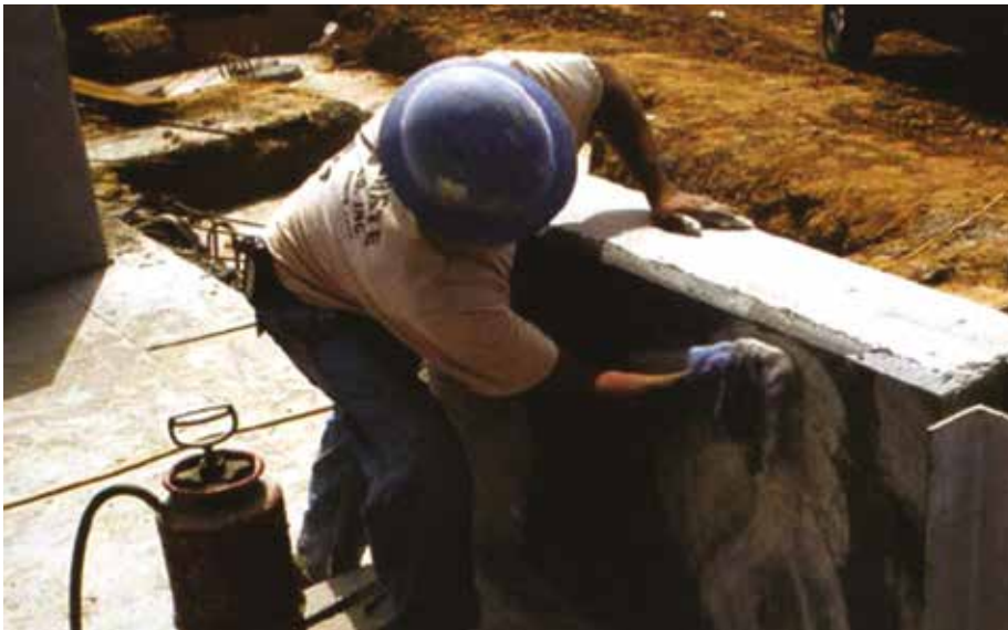
Old methods of sacking and patching required laborious rubbing and meant visual uniformity of results could be difficult. After wetting the wall with a cement slurry, laborers had to rough a silica sand/cement mixture against the wall and rub it into the surface.
