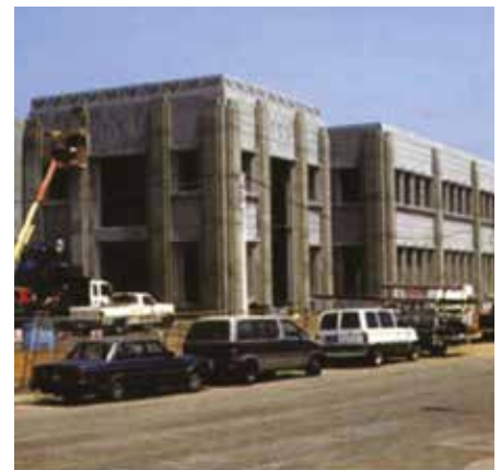
A Santa Fe, California, tilt-up concrete warehouse project comprising a two-story office and a high-bay structure relied on the abilities of new patching compounds to ensure a smooth finish.
