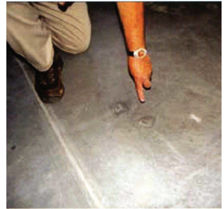
Defects in the floor slab will transfer onto the surface of a tilt-up wall panel—even after attempts have been made to repair the floor. This photo shows a caulked control joint (by foot), patched holes left by fasteners used to install formwork (under finger), and residue from sealant that had been used between formwork and floor slab (across bottom of photo).
