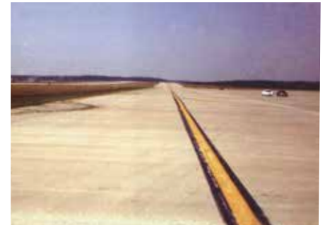
Fig. 8 – After 10 years of use, the airport administration reports that the post-tensioned slab has needed only minimal maintenance.
