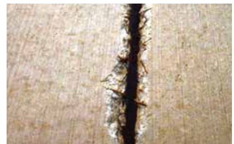
Fig. 10 – The fibrous slab also suffered spalling at its sawcut joints..
