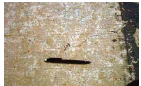
Fig. 11 – The post-tensioned pavement has cracks, but they are tight and less vulnerable to impacts that cause spalls.
