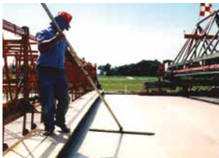
Fig. 6 – Bull-Floating Concrete.
