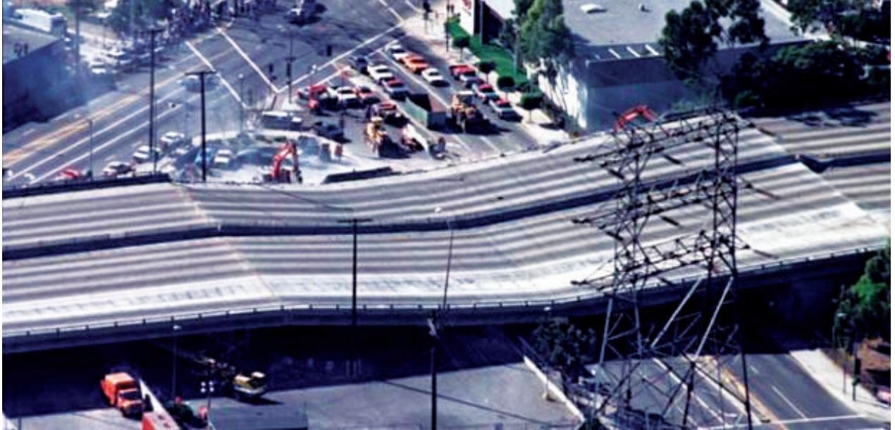
Rapid Set® Cement and Flowable Fill, I-10 freeway (Northridge, CA)
