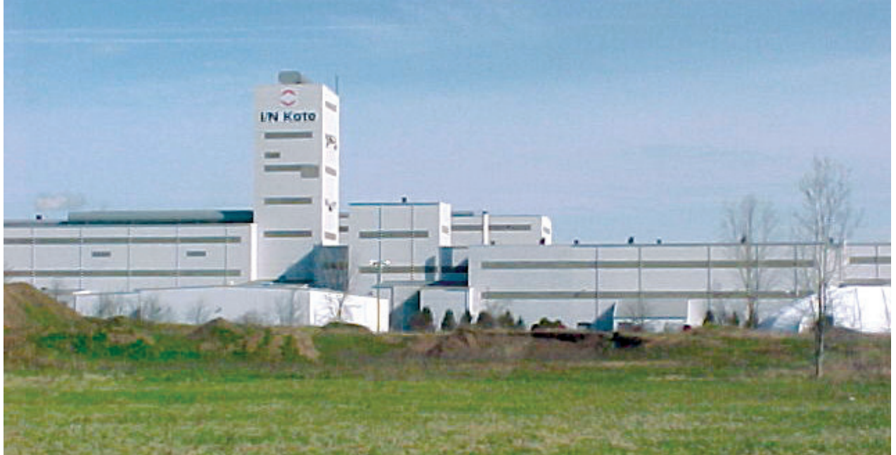
Rapid Set® UltraFlow® 4000/8, Intek/Inkote steel compressor and pump installation (New Carlisle, IN)
