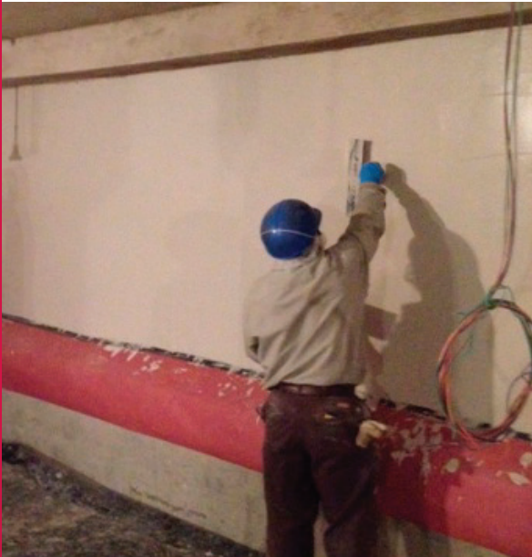
Coast Packing Company Cooler Room
