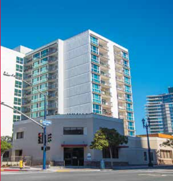
Rapid Set® Eisenwall, San Diego Square (San Diego, CA)
