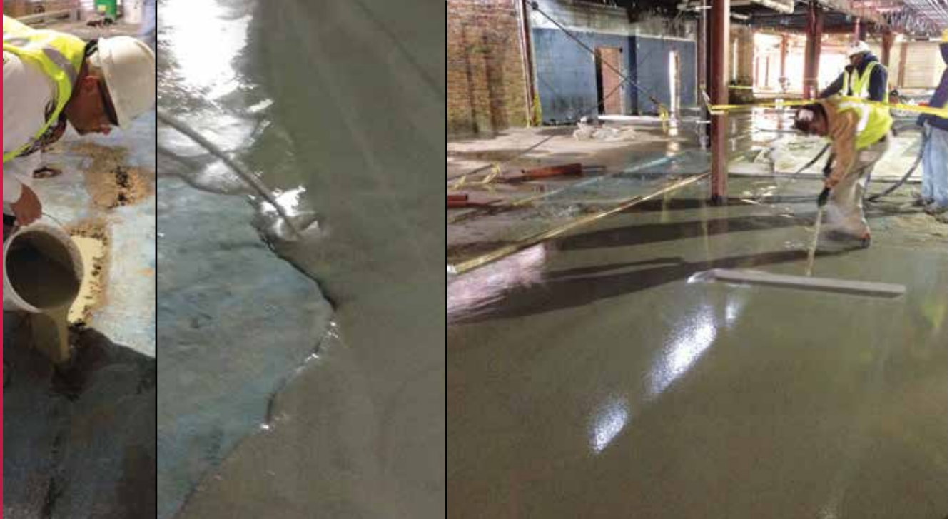
Rapid Set® LevelFlor®, Ft. Jackson Army Training Center (Columbia, SC)
