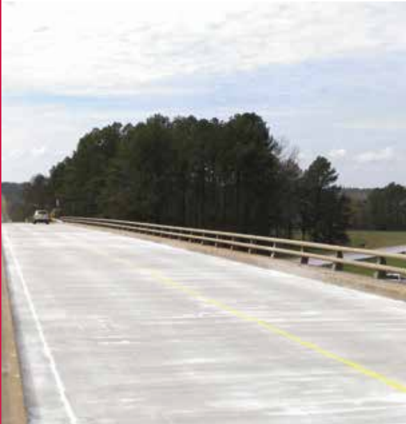
Rapid Set Cement, Route 150 over I-20 in Georgia
