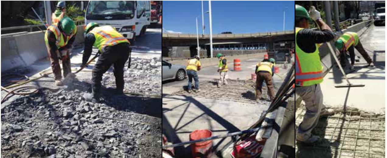
Rapid Set® DOT Cement & Concrete Mix GW Bridge ramps (NY, NJ)
