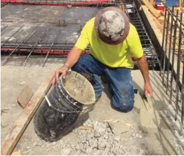
Working Rapid Set® Cement All® deep inside the pores increases adhesion and prevents delamination.
