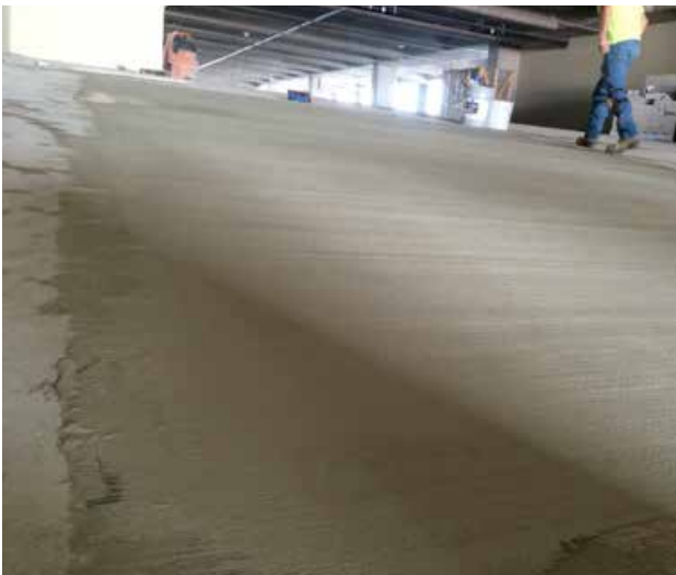
A sponge rubber float was used to apply a broom-like finish.
