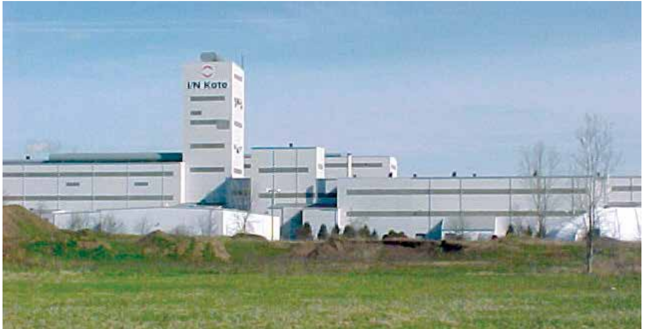
Rapid Set® UltraFlow® 4000/8, Intek/Inkote steel compressor and pump installation (New Carlisle, IN)
