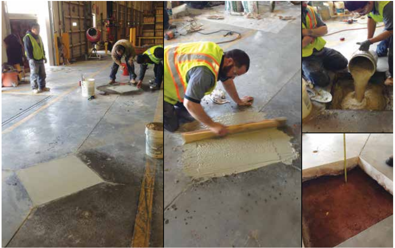
Rapid Set® Concrete Mix, John Deere Distribution Center (McDonough, GA)
