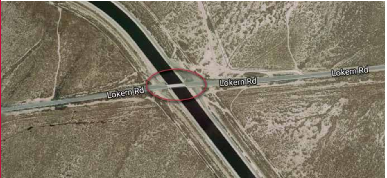
The remote Lokern Road Bridge
