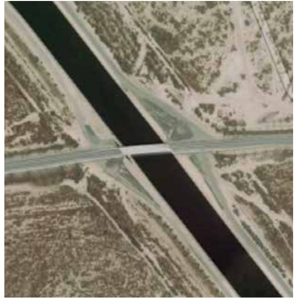
Lokern Road Bridge
