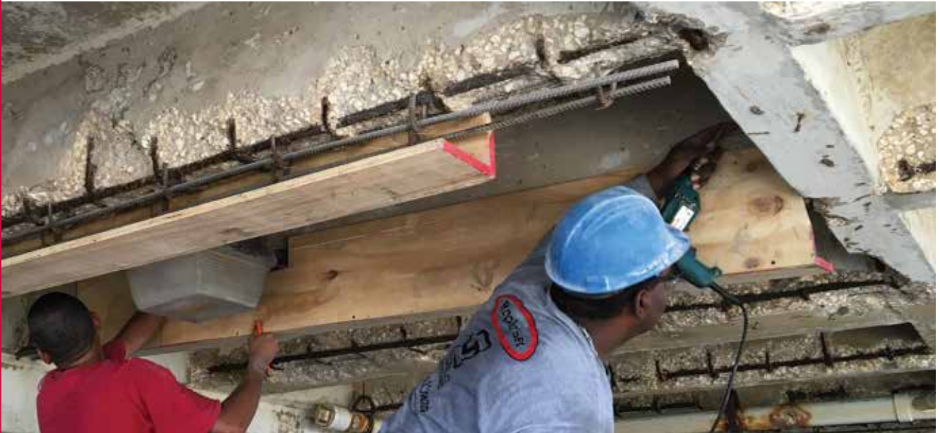
National University College, Arecibo Campus Parking Structure
