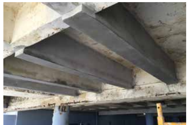
The repair material is ideal for vertical and overhead applications.
