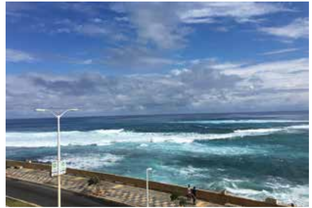
The campus sits 50 feet from the Atlantic Ocean and is subject to strong winds and corrosion
