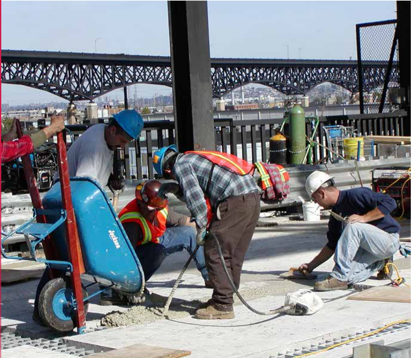
Rapid Set® Cement All® I-93 Bridge (Concord, NH)
