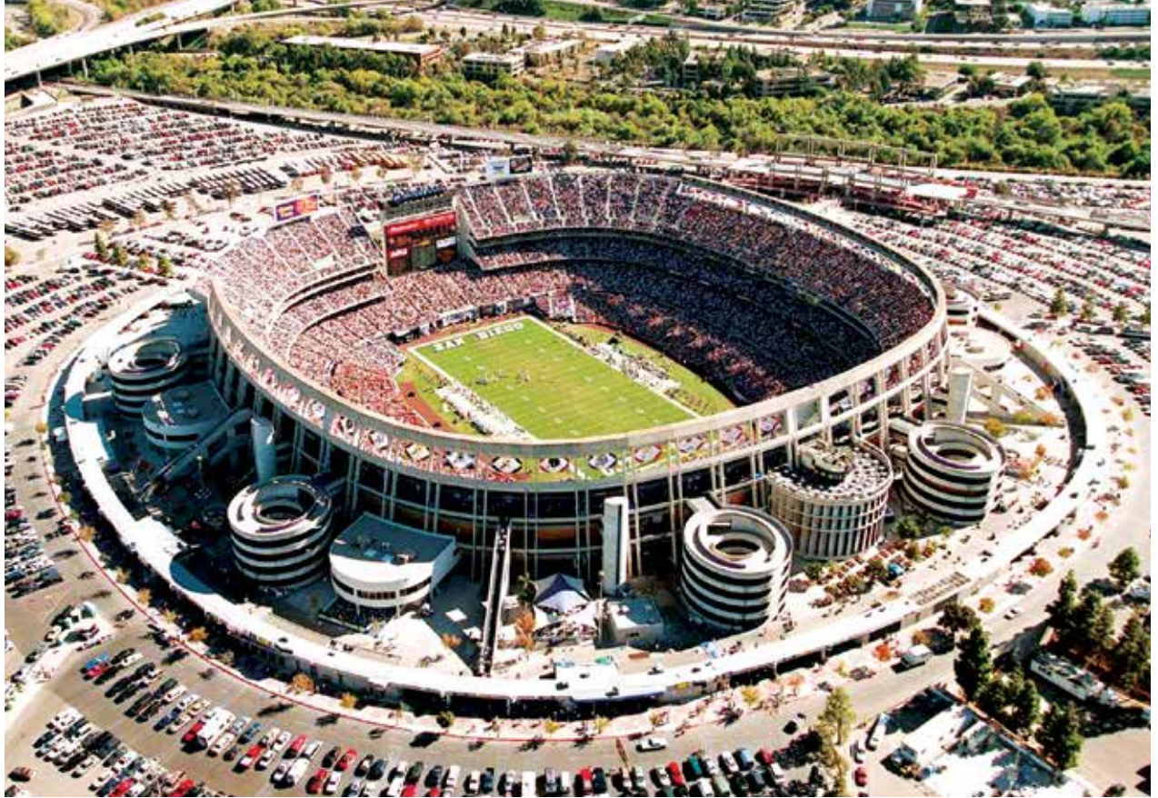
Rapid Set® core products, Qualcomm Stadium (San Diego, CA)
