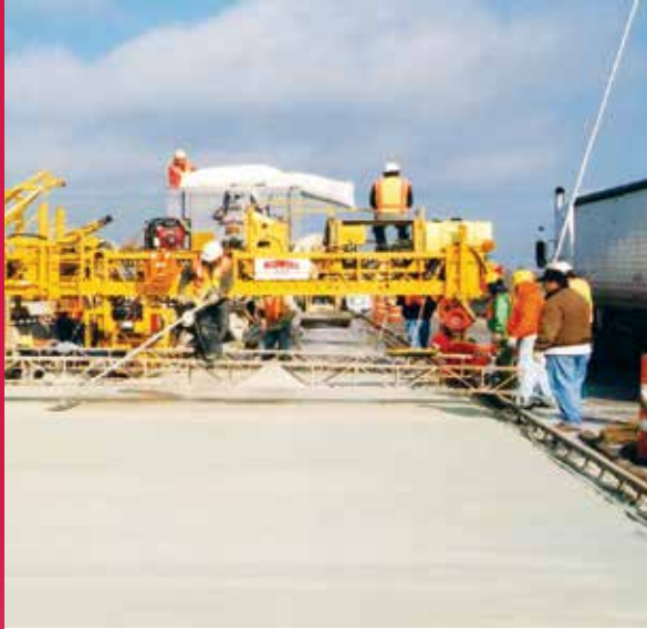
Rapid Set® Latex-Modified Concrete, S.C. Highway 11 (So. Carolina)
