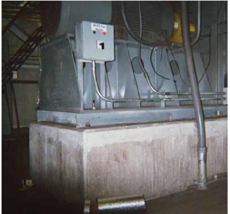
Rapid Set® UltraFlow® 4000/8, USX Boiler House Fan (Gary, IN)
