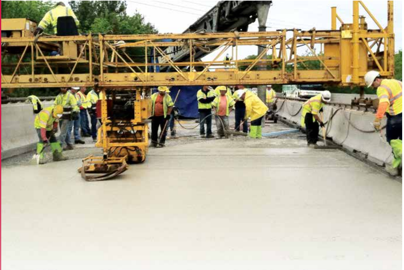
Rapid Set® Low-P™ Cement and Fly Ash, Route 95 Bridge (Foxboro, MA)
