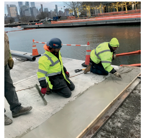
Fixing elevation differences at the Pier in Harsimus Cove
