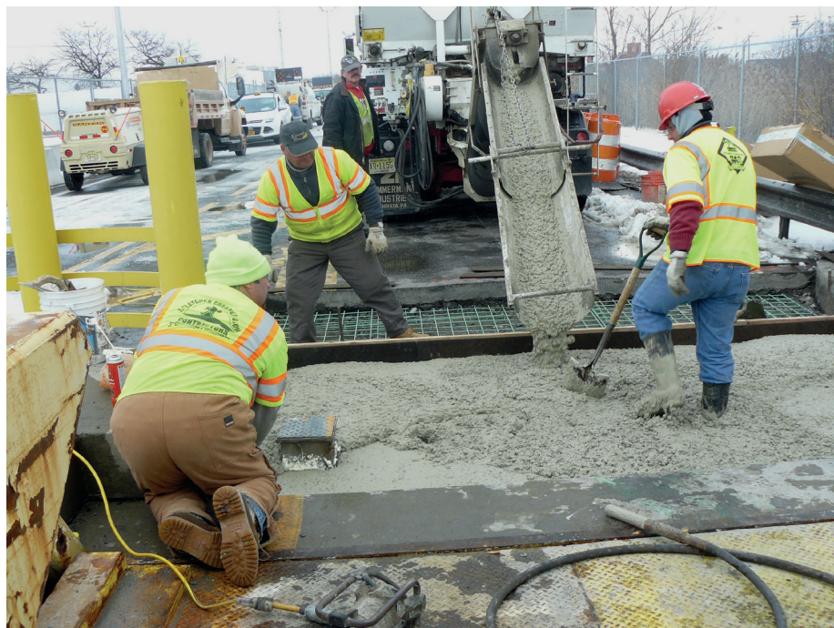
Slab replacement on route 31
