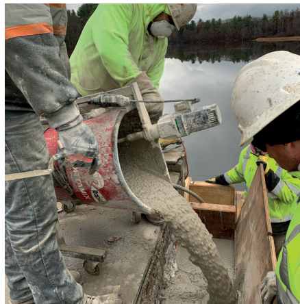
Pouring heated DOT Concrete mix on Salem End Road Bridge
