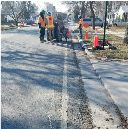
CTS Flowable Fill used to fill micro-trench for Google Fiber
